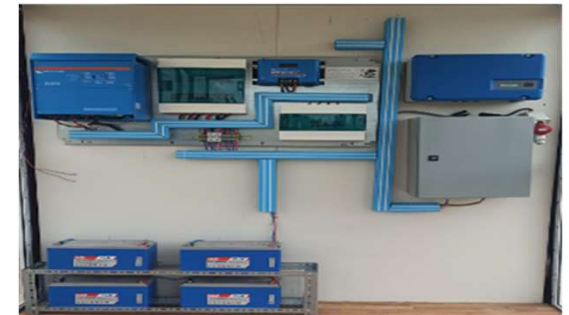
PV controller, inverter and batteries
